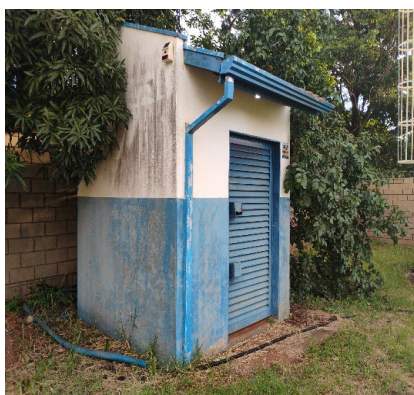
POCO QUEBEC - PAINEL ELETRICO
