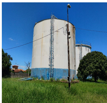
RESERVATORIO R3 - RESERVATORIO APOIADO
